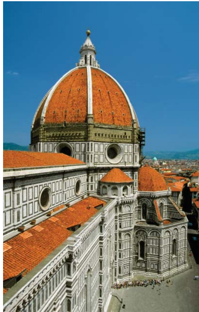
FIGURE 1. The Duomo, the Cathedral of Santa Maria Del Fiore, is a story of human innovation and what might today be called engineering design, but not one of establishing scientific understanding of architectural principles.
